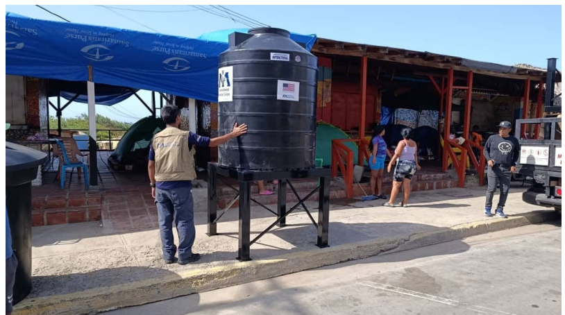
International Medical Corps' WASH team installs a 2,000-liter tank at a transitional camp in La Guaira to safely store clean drinking water for the displaced.
