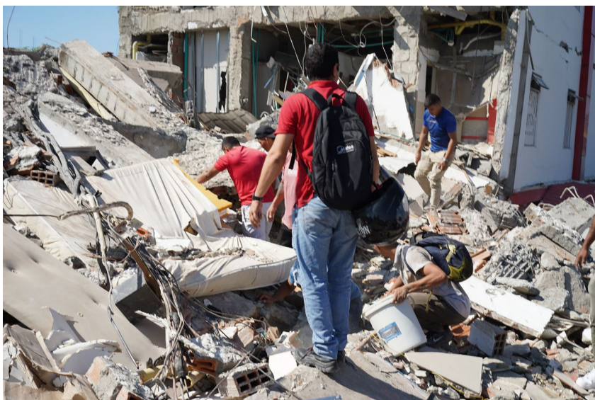
Community members sort through damage caused by the 7.4-magnitude quake. Source: Imago via ZUMA Press
