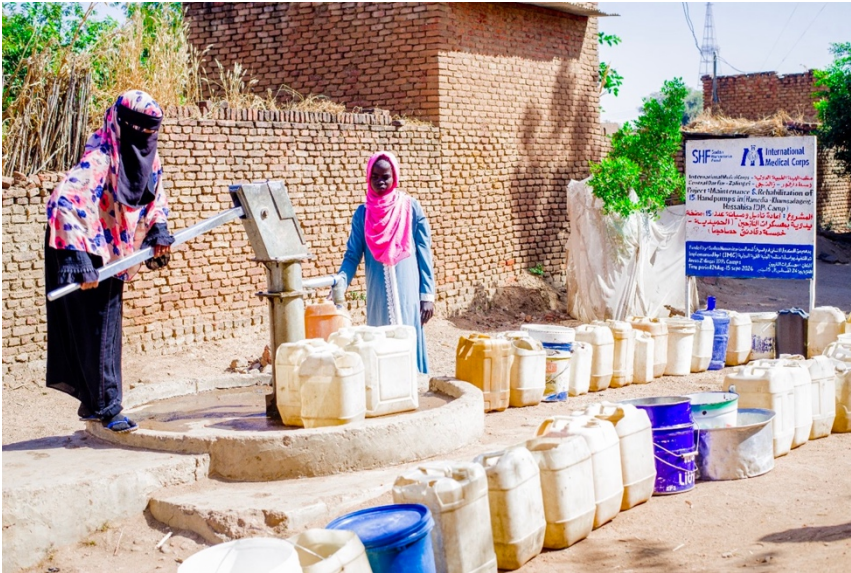
A rehabilitated water point in Hamadiya Camp provides safe water for internally displaced families.
