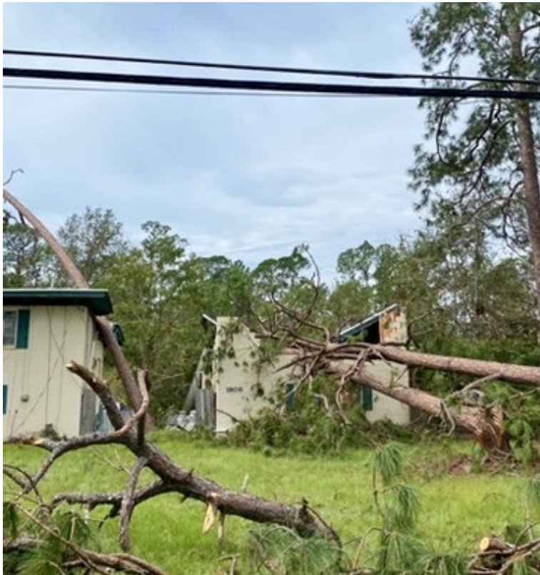
Downed trees and damaged buildings in Lowndes County, Georgia.
