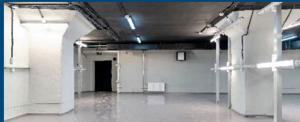
Before-and-after images of the major refurbishment work that International Medical Corps completed on the main bomb shelter beneath Odesa Central Regional Hospital.
