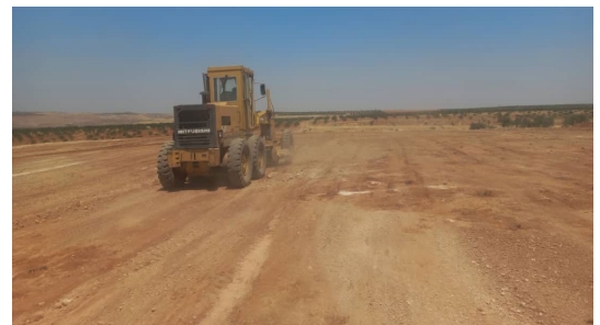
A Hama governorate vehicle prepares ground before installation of nearly 8,000 square meters of solar panels.
