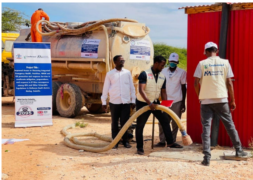
International Medical Corps staff desludging latrines at an affected IDP camp in Galkayo.
