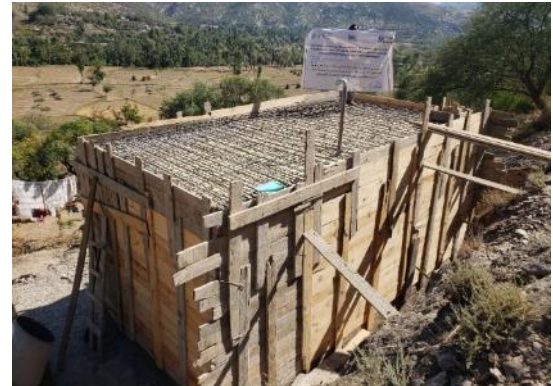
A pipe system under construction in Kunar province.
