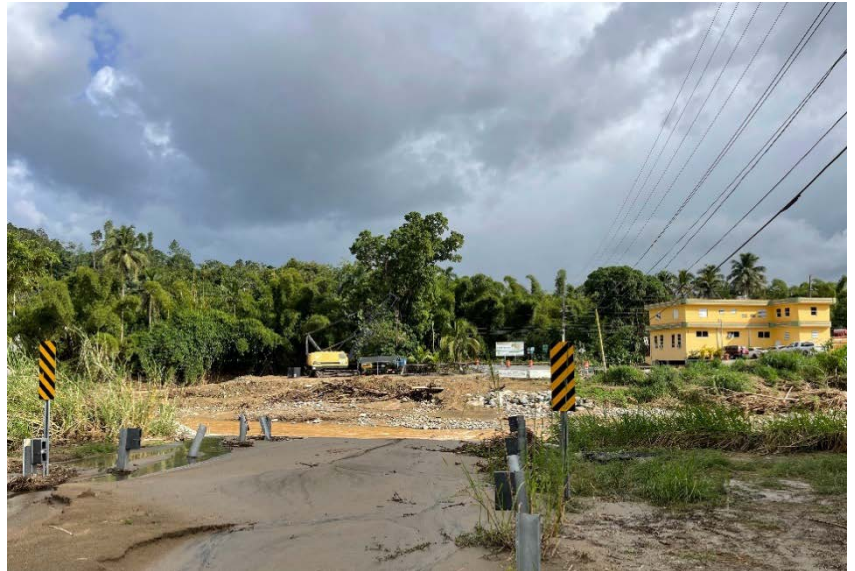
A road beside the Guaonica River in Utuado, Puerto Rico, where a bridge that was swept away by the floodwaters used to be located.
