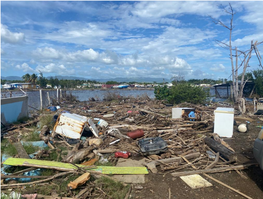
Destruction caused by Hurricane Fiona in the municipality of Salinas, Puerto Rico.
