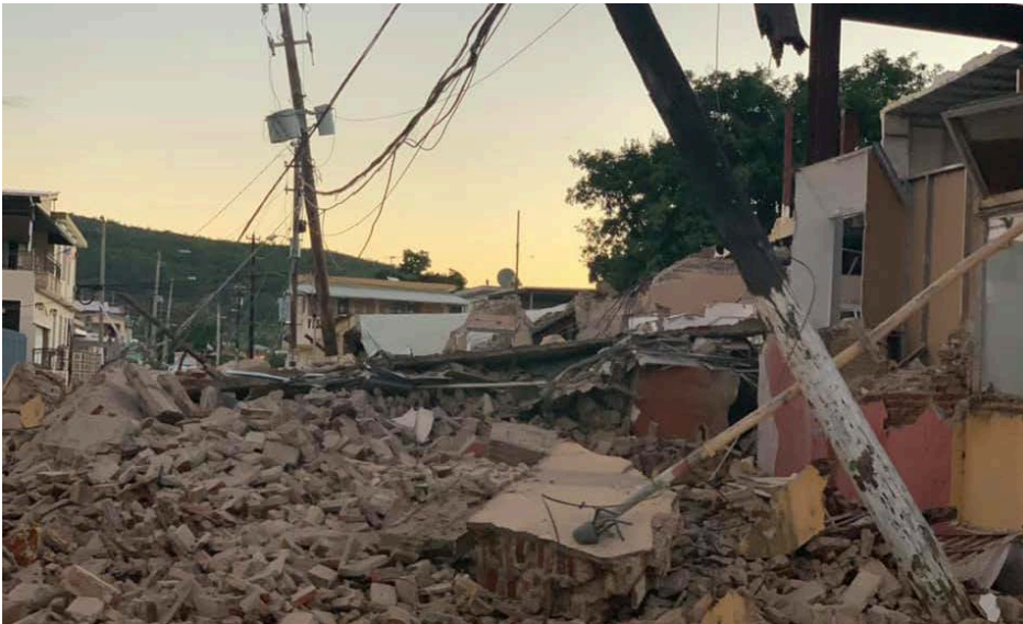
Building and power infrastructure damage early Tuesday morning Guanica, Puerto Rico.
