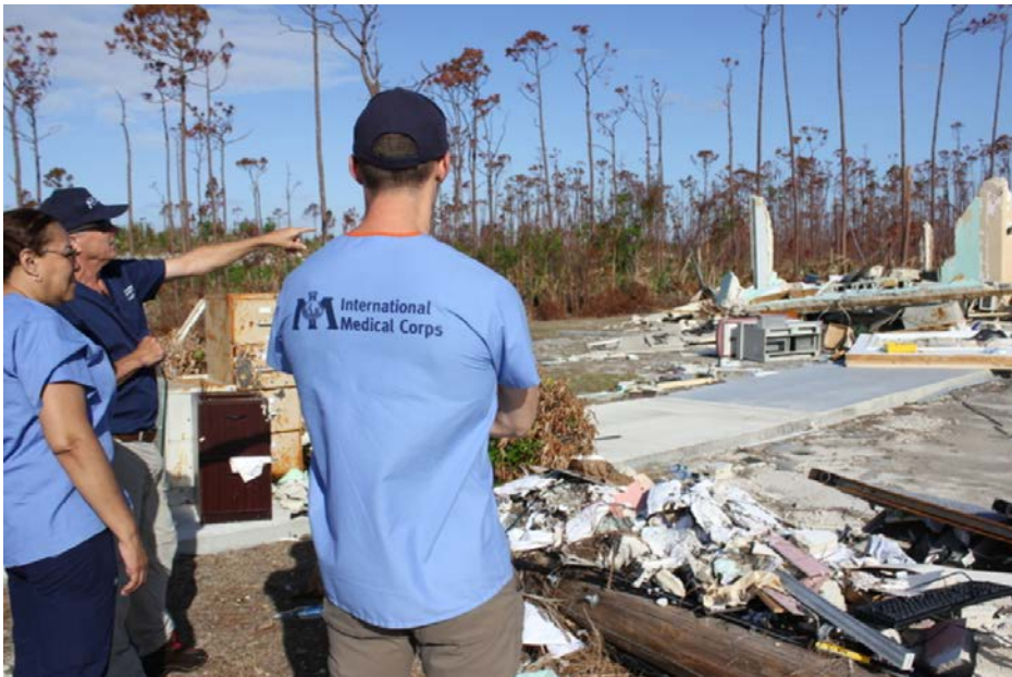
Medical volunteers survey devastation of the health facility in High Rock, Grand Bahama, following Hurricane Dorian.
