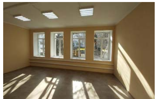
Mykolaev Maternity Hospital, before (top) and after completion of refurbishment.
